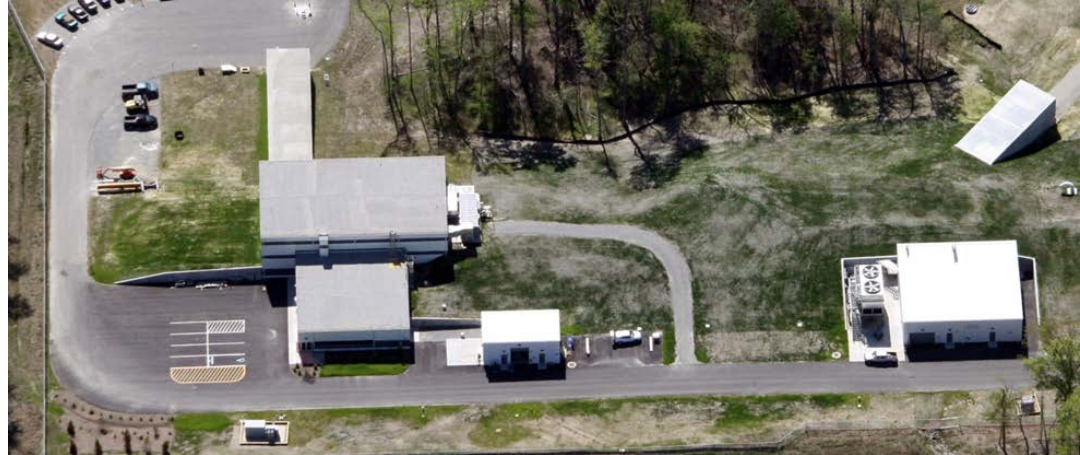
Hall D Complex
