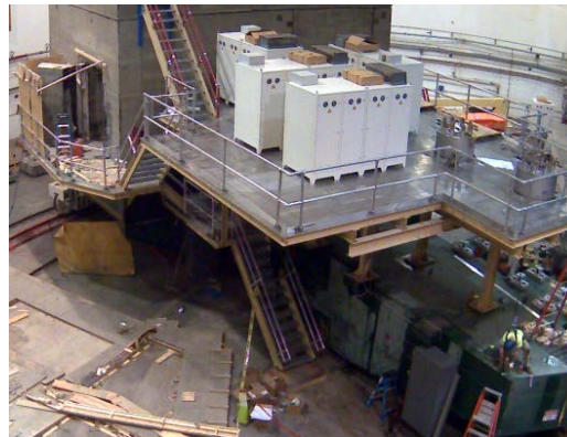
Hall C 77% complete:
