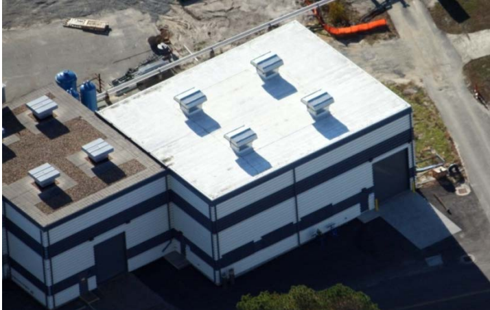
CHL Building Addition
